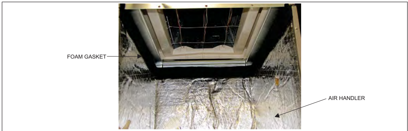
FIGURE 4: Gasket Location
